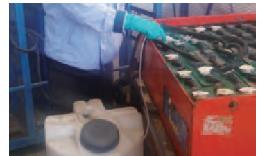
Replenishing water for batteries
