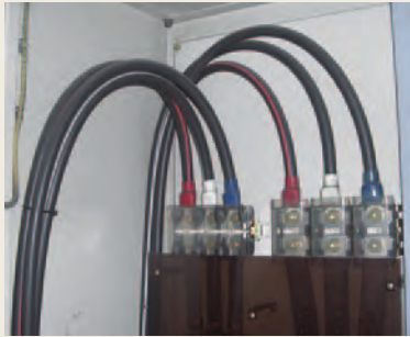
Time-consuming wiring work within the power distribution board
