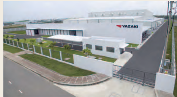
Full view of new Vietnam electric wires factory
