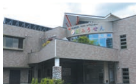
Care Center "Kamifusen" (Susono City, Shizuoka)
