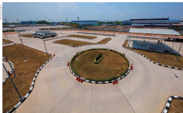
TPRO, Traffic Safety Education and Training Center
