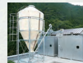
Wood pellet-fueled Araoce*4 installed at Yusuhara Gakuen (municipal elementary and junior high school)
