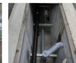
Underground plumbing with a trench structure
