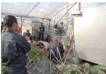
Installation of a fan heater
