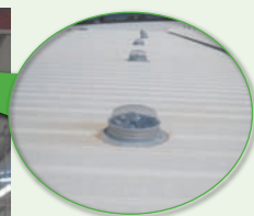
Solar tube supplies sunlight to illuminate the factory.
