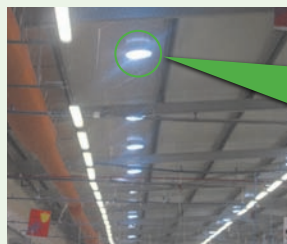
Solar tube supplies sunlight to illuminate the factory.
