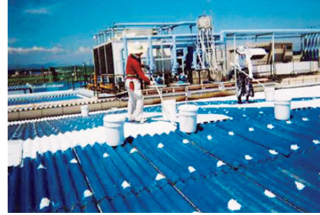
Painting the roof with heat blocking paint (Ohama Factory)
