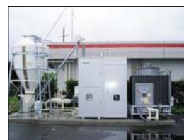
Aroace wood pellet-fired double effect absorption chiller-heater 10RT (35kw cooling capacity) Yakushima model
