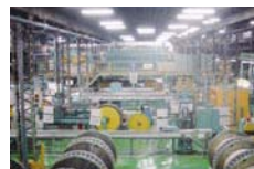
High-efficiency fluorescent light bulbs in the Numazu Factory
