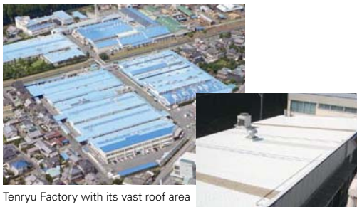
Roof painted with white heat-shielding paint
