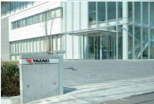
Entrance to Shizuoka Branch, built to barrier-free design
