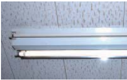
Lighting that uses a dummy tube and a reflector
