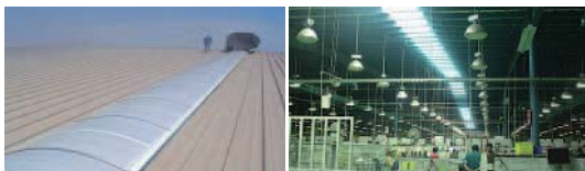
The dome-shaped sky roof installed above the final assembly line
