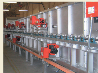
A large continuous kiln manufactures Eco-Pumice
