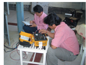
TYE employees inspecting and repairing electric cables in Phuket
