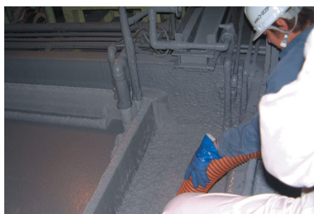
Replacing paint in an electrodeposition tank at the Hamamatsu Factory
