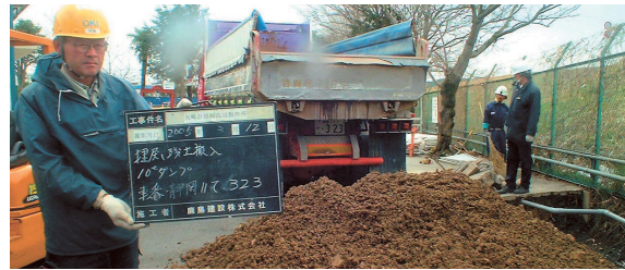
Soil replacement at the Shimada Factory
