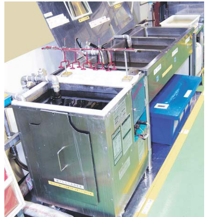
Alkaline cleaning solution filtration device at the Haibara Factory
