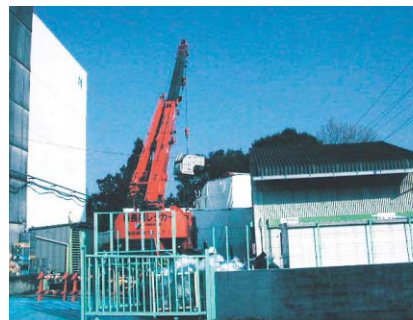
Incinerator removal in progress at the Haibara Factory
