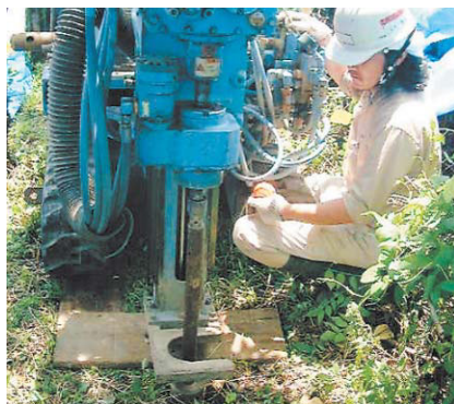
Soil boring to check for dioxins
