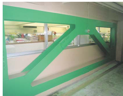
Reinforcement construction at offices and factories
