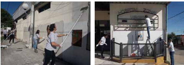
Employees repairing the exterior walls of a hospital
