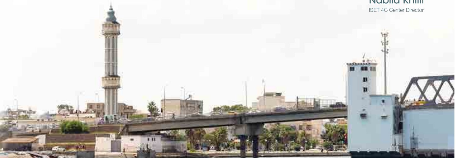
A bridge spanning a canal in Bizerte city
